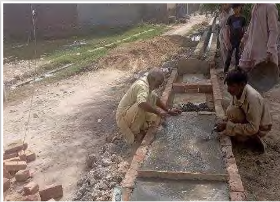
Construction of Drain Okara Cantonment Board
