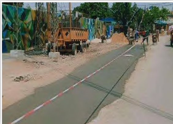
Laying of sewerage lines from Cantt Board office to Magnum Mall Civil Lines
