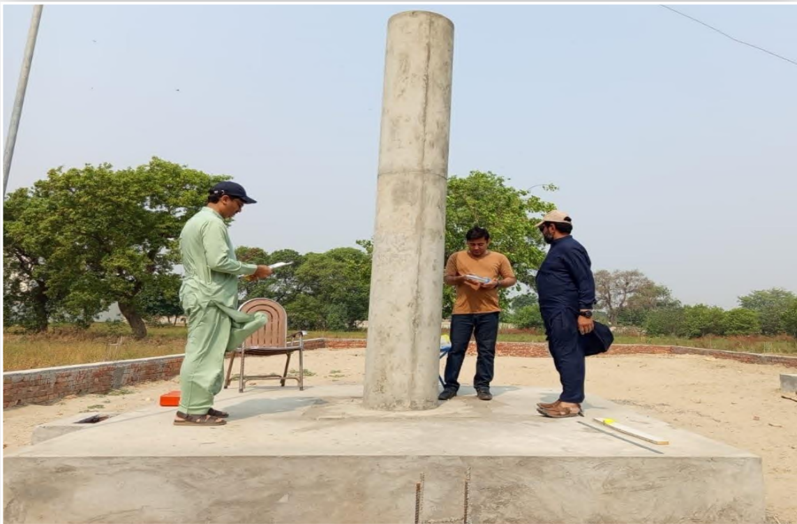
Mr. Muhammad Arshad (Director Technical and coordination, Sop) along with QC Team conducting inspection of newly constructed CORs Station at Lahore.
