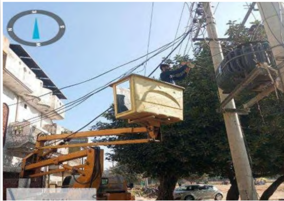
Installation of LED Lights at Rahwali, CB Gujranwala
