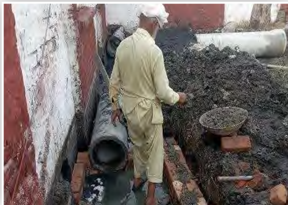
Laying of Sewerage Pipeline at Koulsar Colony, Hyderabad Okara Cantonment Board
