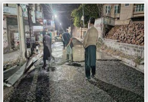
Construction of PCC Street at Kholy choona Kari Ward No. 4, Abbottabad Cantonment Board
