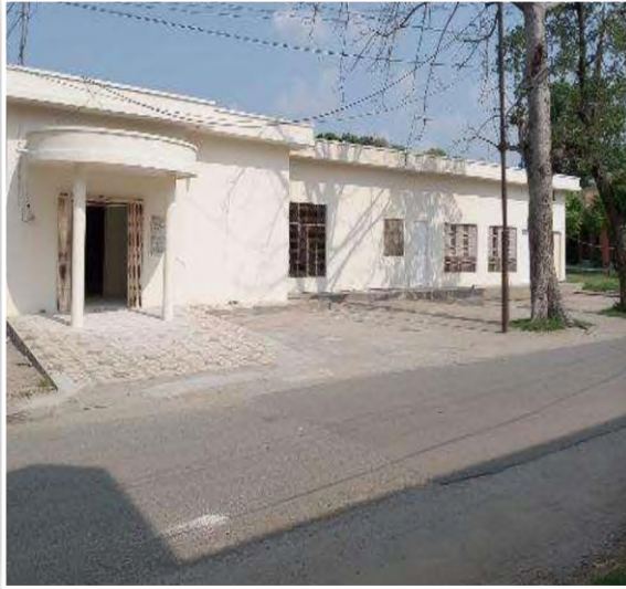
Renovation of Civic Centre, CB Gujranwala
