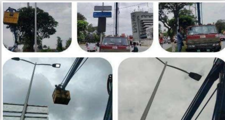
Repairing of Street Light Rawalpindi Cantonment Board
