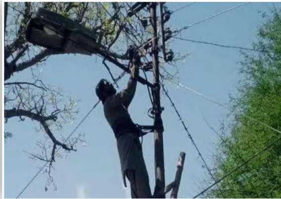
Repairing of Street Light D.I Khan Cantonment Board
