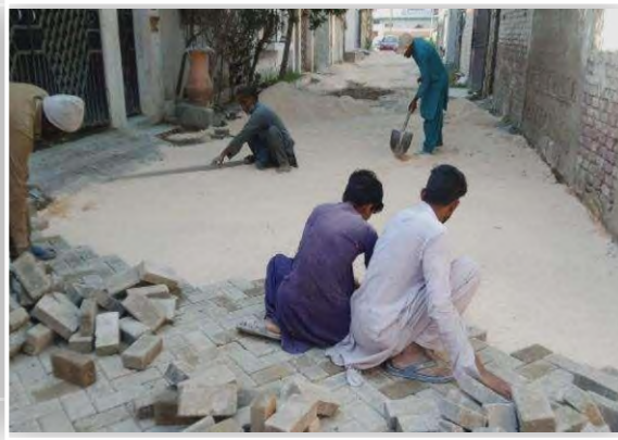
Tuff Tiles Work at Hyderabad Cantonment
