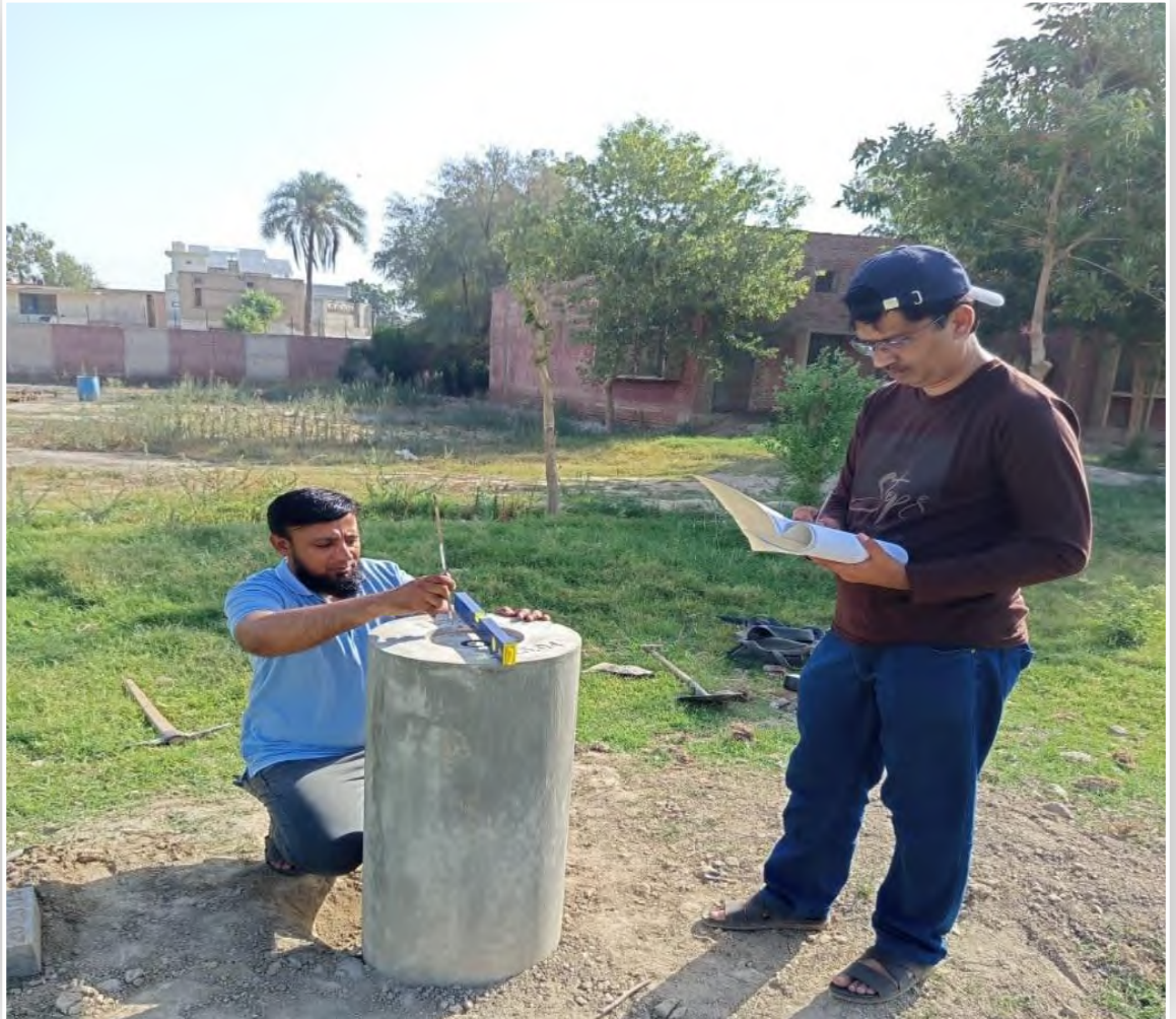
QC Team during inspection of newly constructed GNSS under Datum Project at Bahawalpur.
