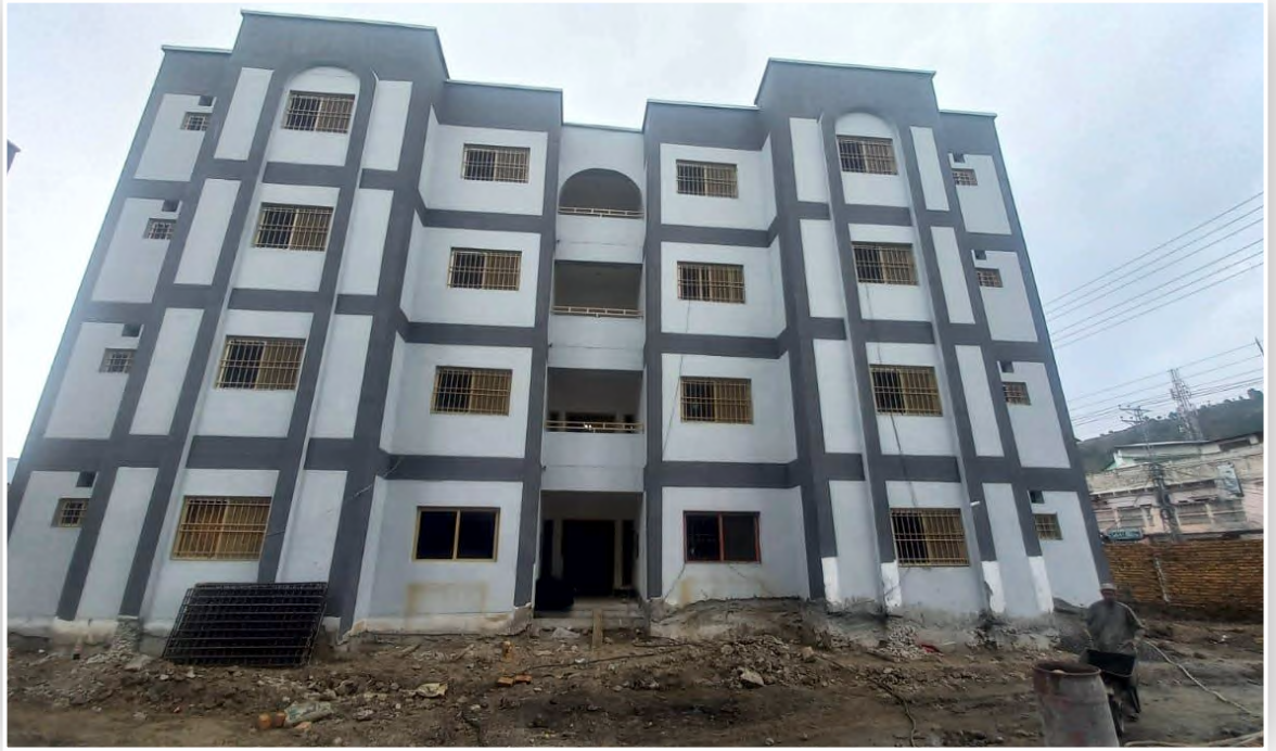
NEWLY CONSTRUCTED FLATS AT PMAD ABBOTTABAD
