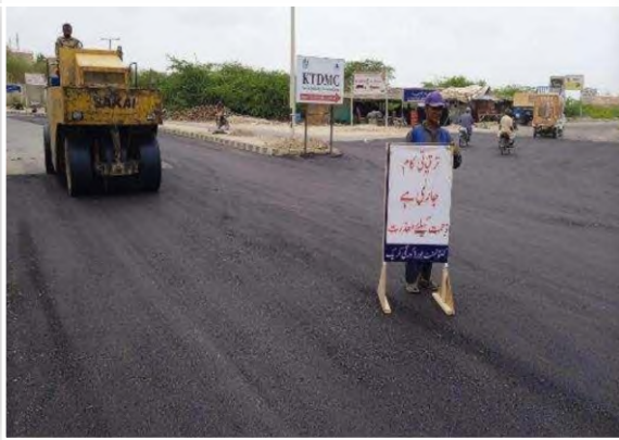
Re-carpeting of Road Korangi Creek Cantonment Board
